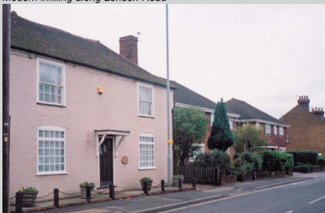
Modern infilling along London Road
