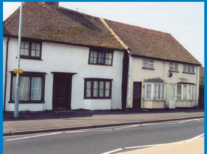
Traditional materials and windows in London Road
